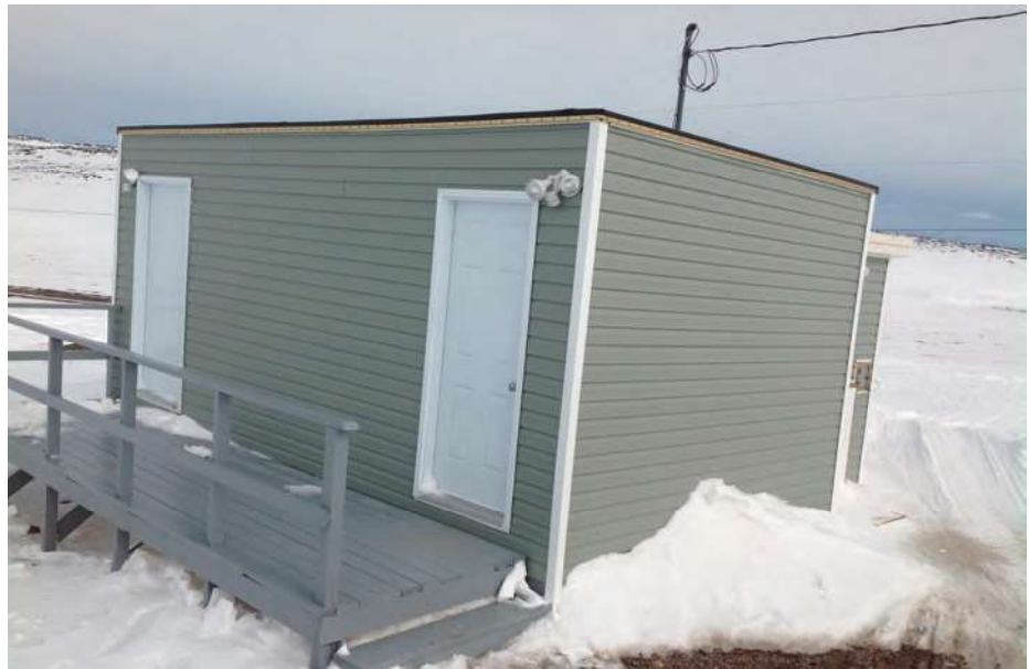
The pump house at Shambler's Cove Pond, Greenspond, NL. Photo credit: Jen Daniels
