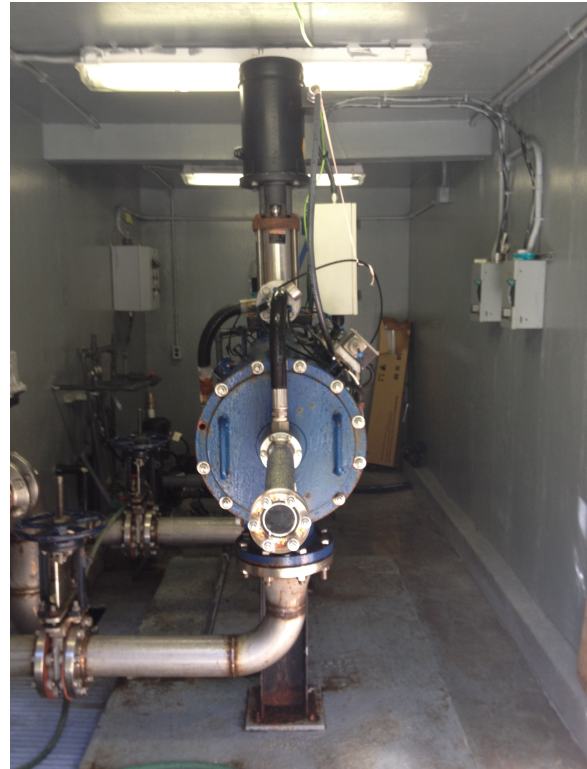
FILTOMAT Filter in the Pump House
